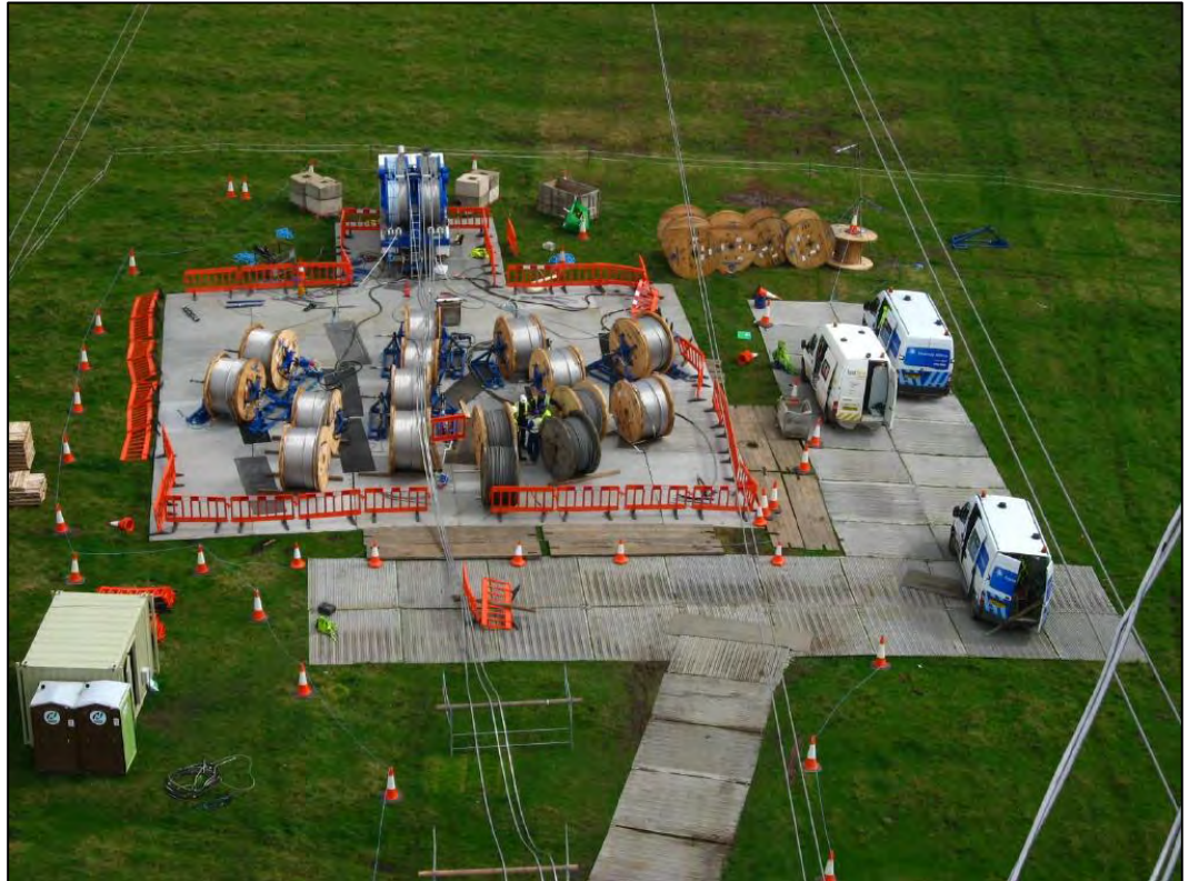
Figure 5.4. Overview of Conductor Winch Position and Drums
