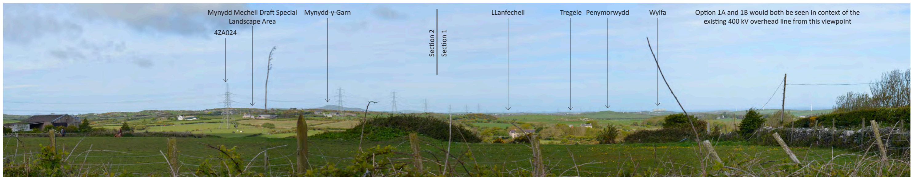
Photo 1.5: View from Four Crosses north-east of Rhosgoch looking west showing existing 400 kV overhead line and Wylfa in the distance
