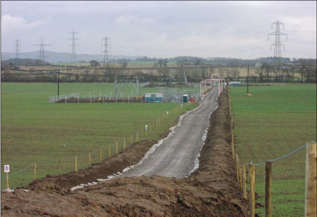
Figure 5.2. Temporary Stone Access Track with Pylon Construction Area
