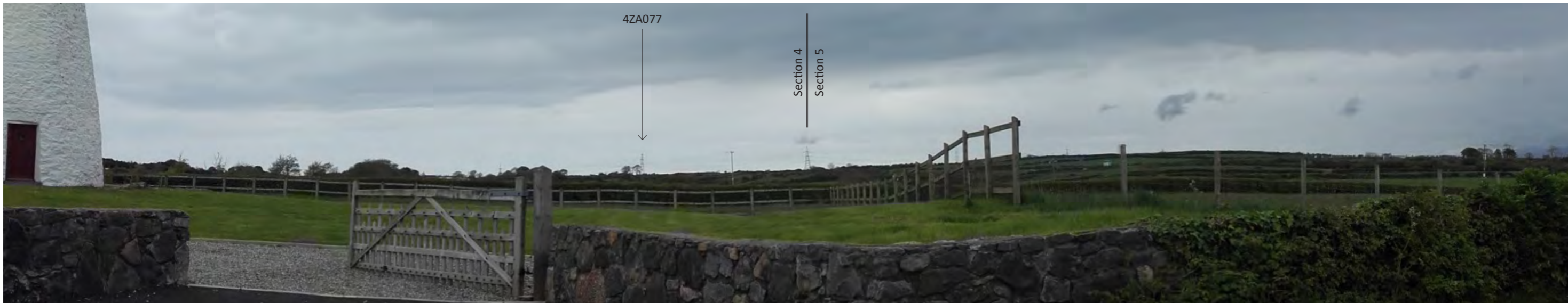
Photo 4.4: View from northern edge of Gaerwen near Melin Sgutha (Union Mill) towards the existing 400kV overhead line on the distant skyline
