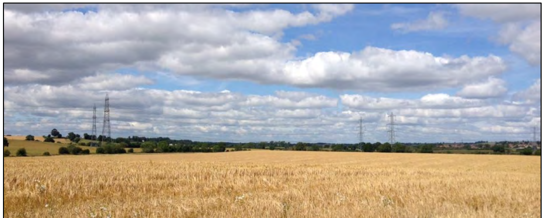
Photo 7.1. Parallel Overhead lines in County Durham.
